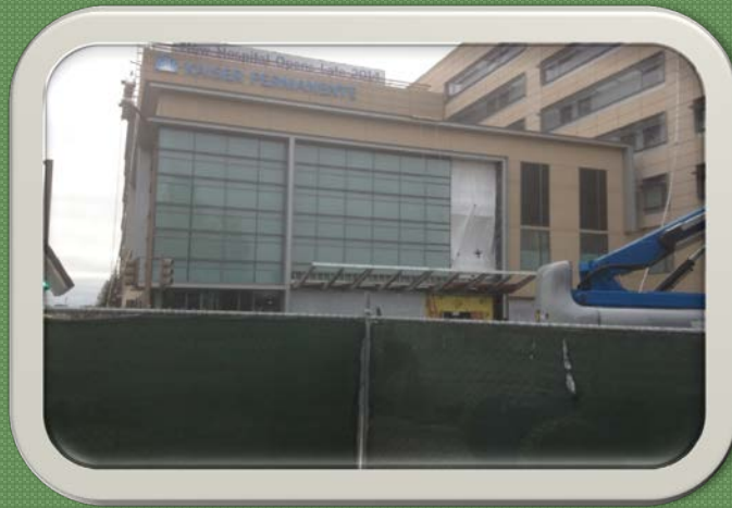
Panels with windows and metal paneling
