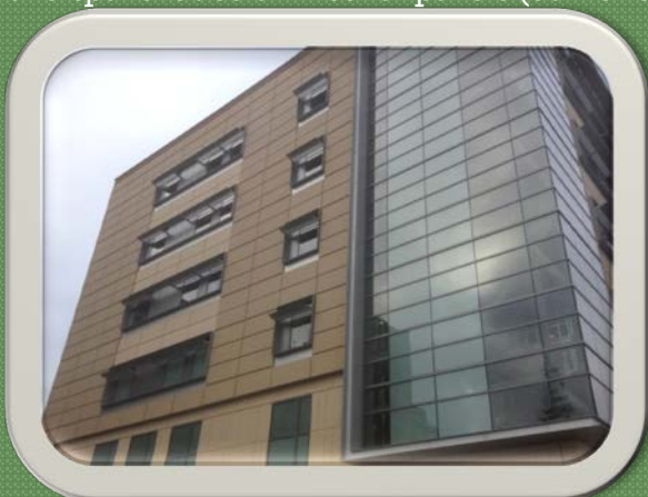
Window box panels adjacent to stair
