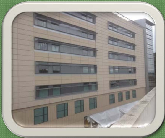
Main elevation with window box panels (lighter color), and spandrel/column cover panels (darker color)
