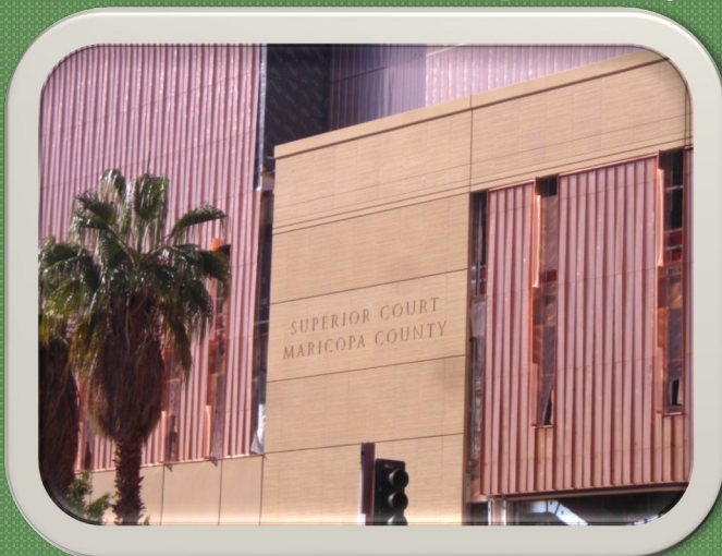
Precast panels with lettering.
