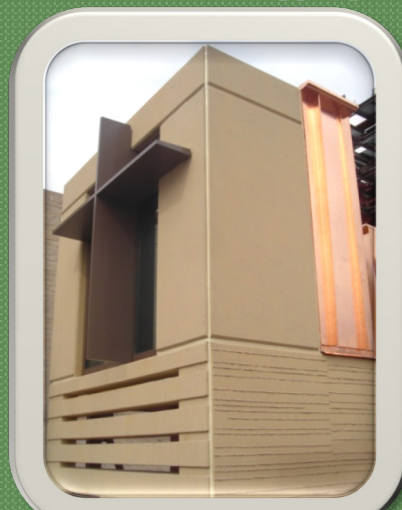
Project mock-up panels. Louver panels at bottom.
