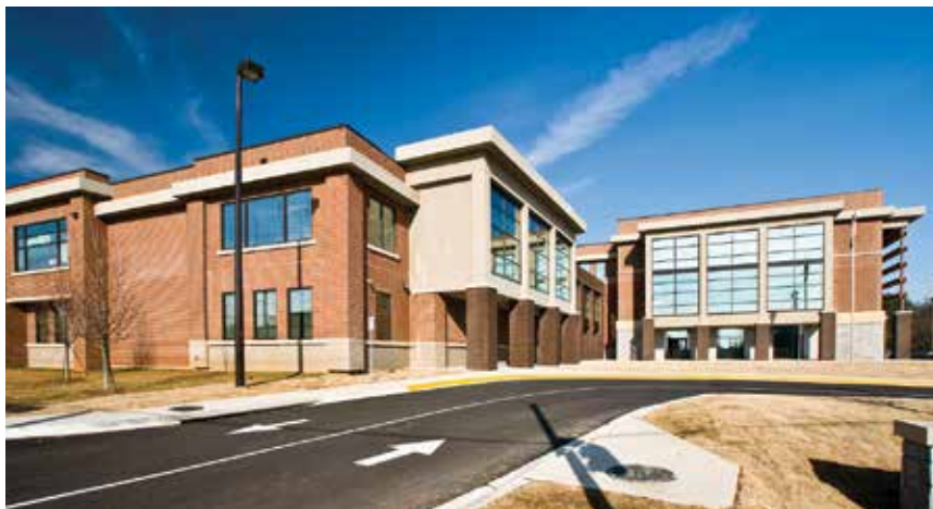
Tucker High School, in Tucker, Georgia, used a total precast system including columns, beams, double-tees, stairs, and insulated wall panels to complete this 340,000 sq. ft. project. Photo credit: Photo courtesy of George Spence, Metromont
