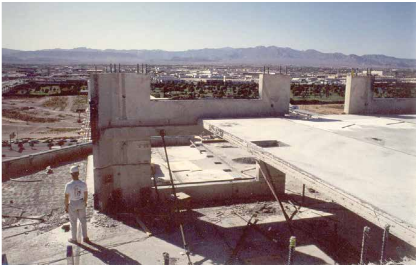
The MGM Grand Hotel and Casino in Las Vegas used a precast concrete structural and envelope system to create the world's largest hotel at that time. Photo credit: Photos courtesy of FDG
